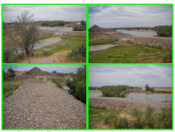
Photo No. 4: Filter berm level was increased to function properly
