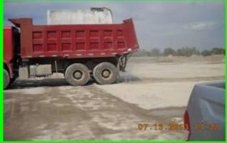
Photo No. 19: Watering to suppress dust at the cement batching plant near the camp
