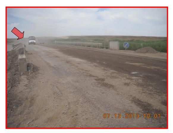
Photo No. 12: Dust generation at the un-watered part of the road
