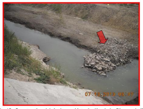
Photo No. 15 : Construction debris dumped into the Karabalta River and affecting flow direction
